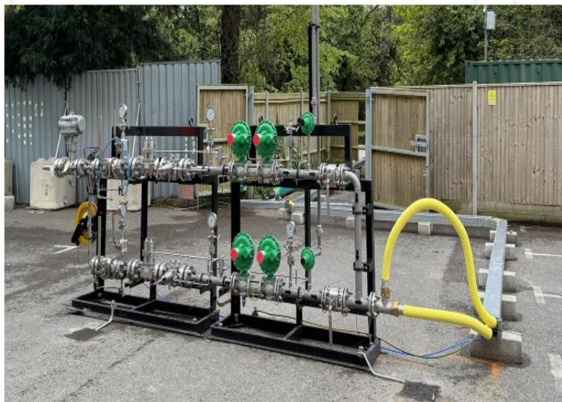
Fig 5: Cremator 3 was completely disconnected from Natural Gas for the duration of the trial. The two NG burners were replaced by hydrogen burners (as seen above). These were then connected to a low pressure hydrogen pipeline, through the pressure reducing station (top right) 7
