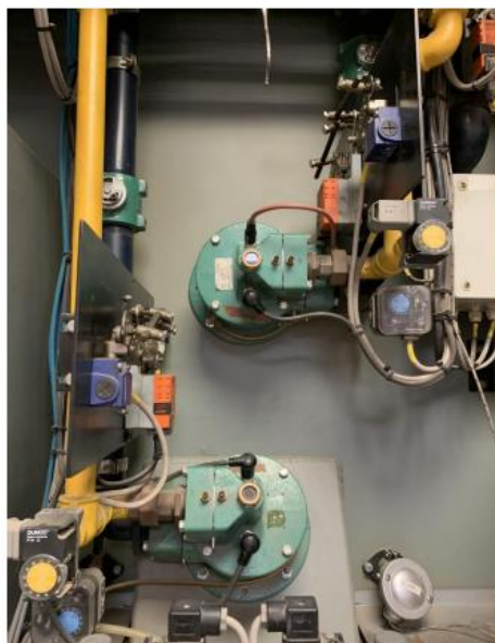
Fig 5: Cremator 3 was completely disconnected from Natural Gas for the duration of the trial. The two NG burners were replaced by hydrogen burners (as seen above). These were then connected to a low pressure hydrogen pipeline, through the pressure reducing station (top right) 7
