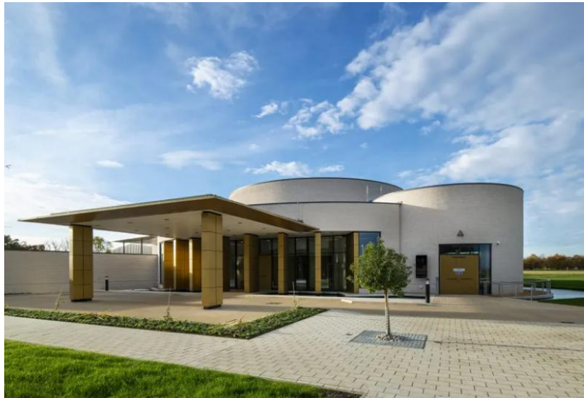
Fig 10: Huntingdon Crematorium, operating on green tariff
